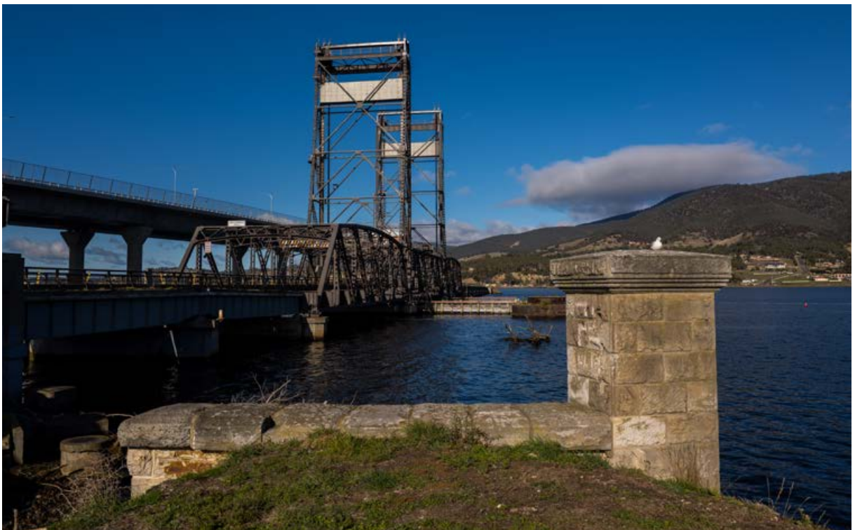
Bridgewater Bridge from the northern embankment. The evolution of transport across the Derwent is demonstrated by the sandstone abutments from the 1893 bridge, the 1946 Road and Rail Bridge and the latest bridge opened in 2025. Credit - Alistair Bett.
