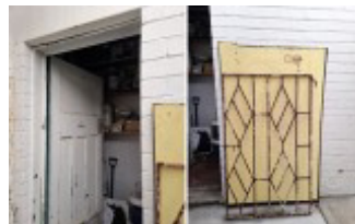
Toilets to rear; iron gate to be restored © NRE 2026
