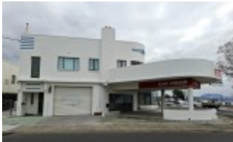
Maning Avenue frontage, looking north-east © NRE 2026
