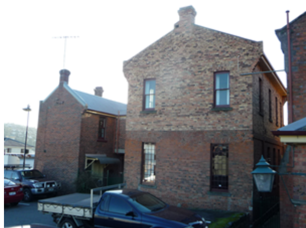
Additions to the rear of Milton Hall ©2013 NRET
