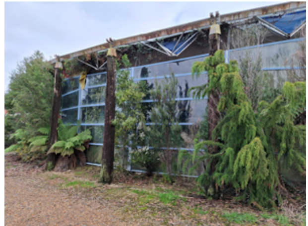
View north-west from the waterfront © NRE 2024
