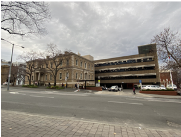
Davey St Wing, Elizabeth Street Heritage Tasmania 2021
