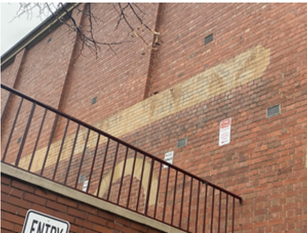
Ghost signage and former windows, wstn elev Heritage Tasmania 2021
