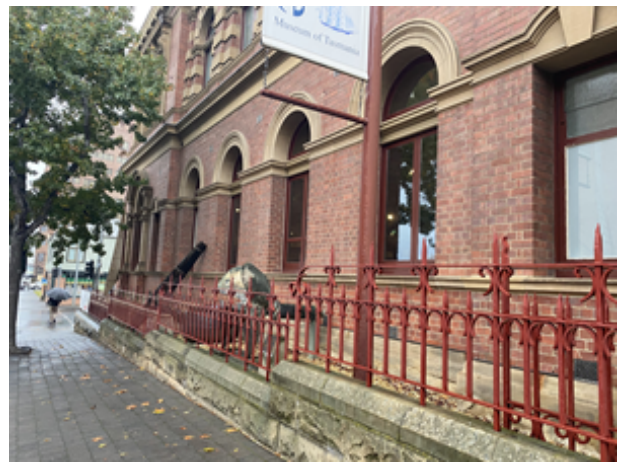
Argyle Street boundary Heritage Tasmania 2021
