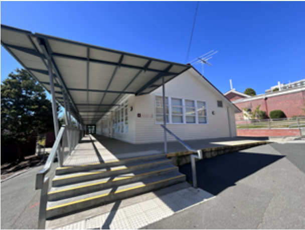
Art and Classroom block, northern elevation Heritage Tasmania
