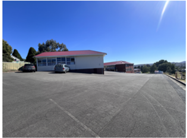
Domestic Arts building and Art and Classroom block, southern elevations Heritage Tasmania
