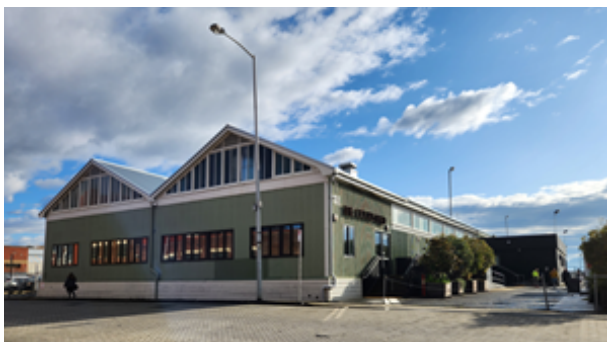
Hobart Railway Goods Shed from south-east on Evans Street. © NRE Tas Aug 2023
