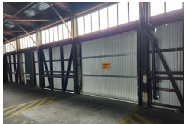
Perimeter walls' alternating braced and unbraced bays indicate the former locations of goods doors. © NRE Tas Aug 2023
