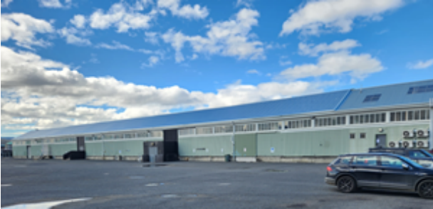
Hobart Railway Goods Shed from the west.
