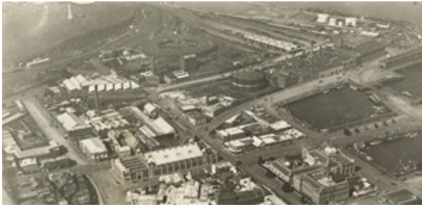
undated but between 1924 and mid-1930s: the long roofs of the Goods Shed are visible at upper right.
