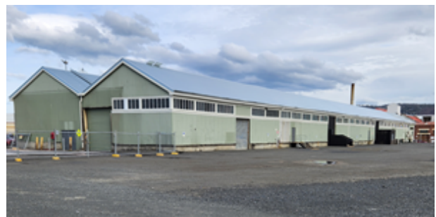
Hobart Railway Goods Shed from north-west. © NRE Tas Aug 2023
