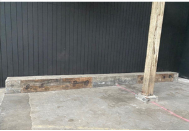
The remnant buffer blocks of board-marked concrete.
