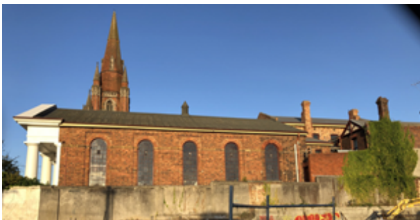
Milton Hall from the west, showing additions at rear ©2025 NRET
