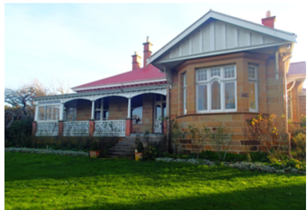
Barton house ©2014 NRET
