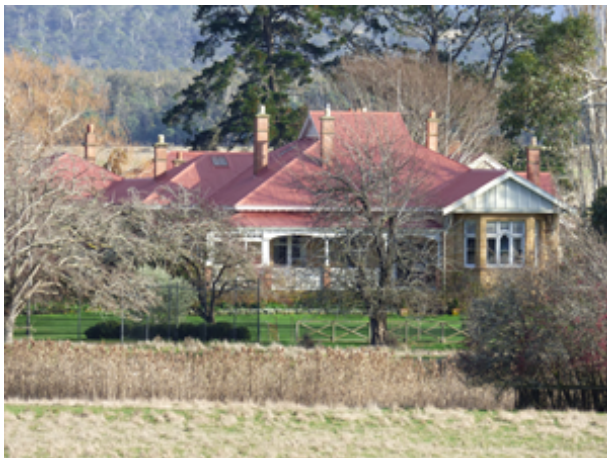
Barton house ©2014 NRET
