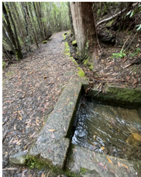
Boxed masonry intake, Milles Track ©2026 NRET
