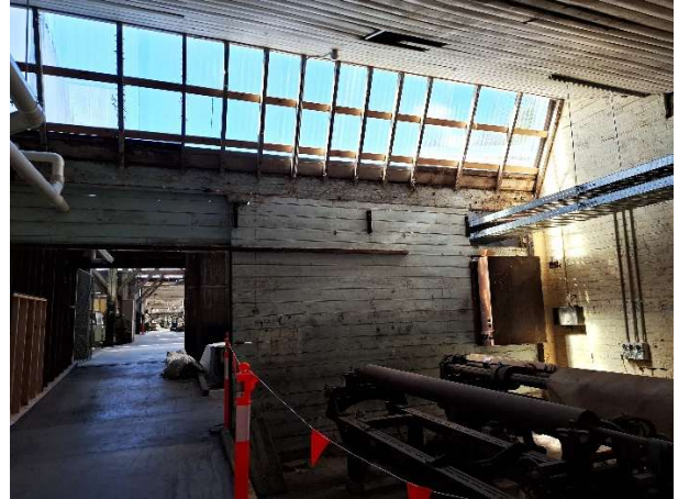
Western wing: timber panelling, disused machinery © NRE 2025
