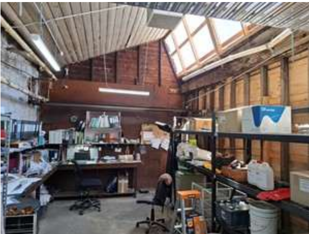
Western wing: central office, timber lining © NRE 2025
