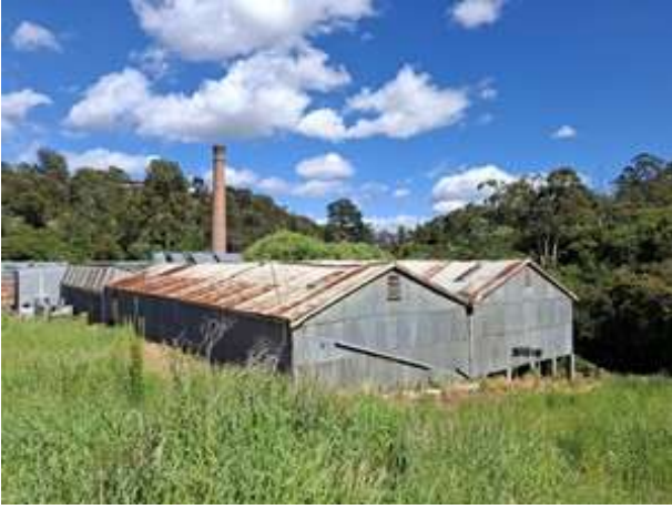
Northern section: from hatchery site, toward creek © NRE 2025
