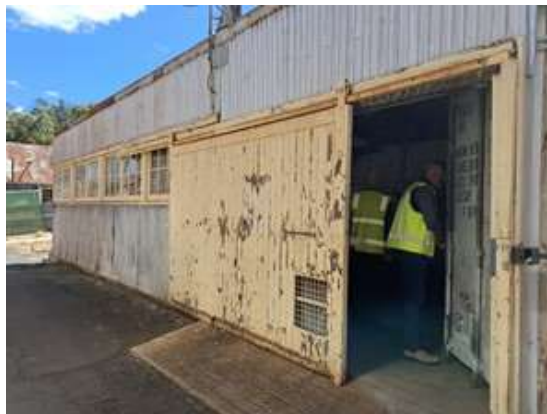
Maintenance shed: from alley © NRE 2025
