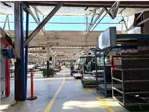
Western wing: finishing section; hybrid structure © NRE 2025
