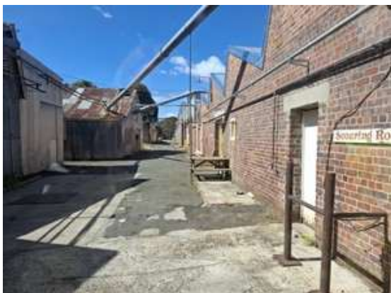
Central alley: from north © NRE 2025
