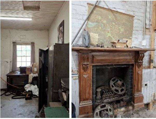
Western wing: front office/ storage areas © NRE 2025
