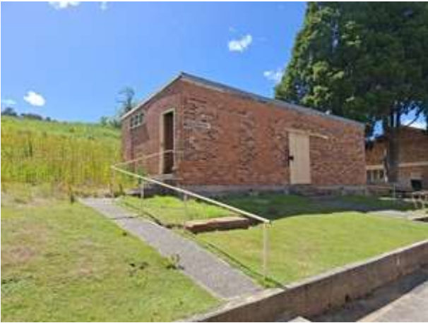
Amenities block: with eastern wing behind © NRE 2025
