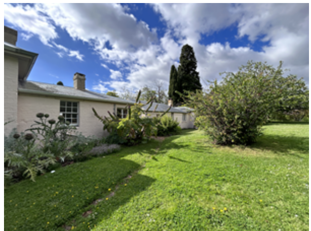
Eastern elevation showing varying forms, building phases 1850s onwards and heights of chimneys Heritage Tasmania
