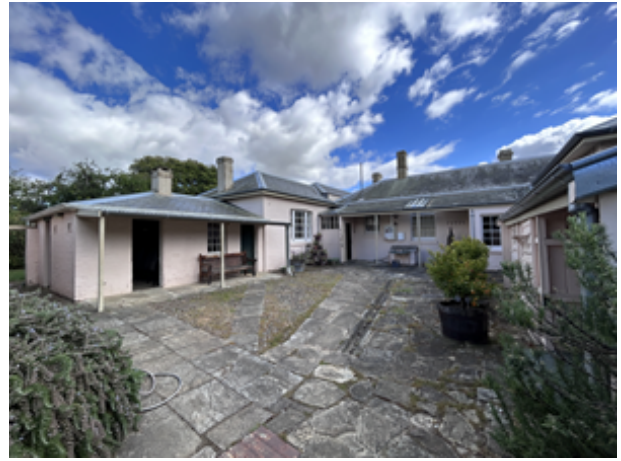
Courtyard behind, including dog kennel Heritage Tasmania
