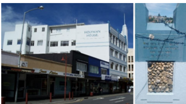
North-western side; Stone from foundation on rooftop ©NRE 2023
