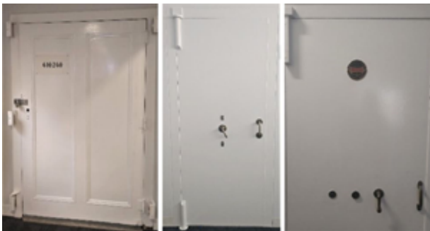
Interior – Strong room doors and door furniture ©NRE 2023
