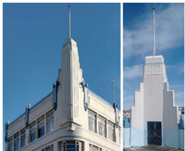
Beacon details – from street; roof top ©NRE 2023
