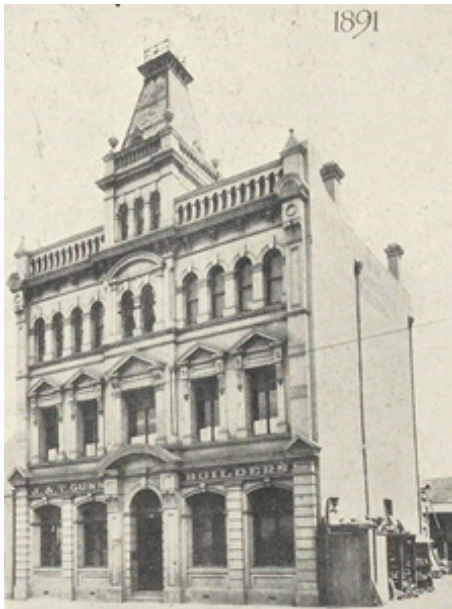
Circa 1892 building - prior to fire Weekly Courier 7 March 1903
