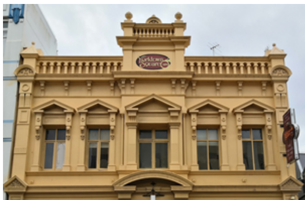
J & T Gunn Building - Brisbane Street façade detail ©NRE 2020
