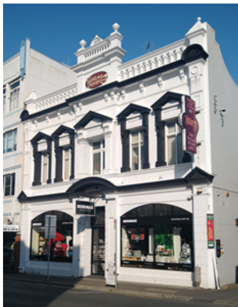
J & T Gunn Building - Brisbane Street façade ©NRE 2023
