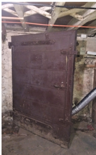
J & T Gunn Building - Basement fire doors and timber floor ©NRE 2023
