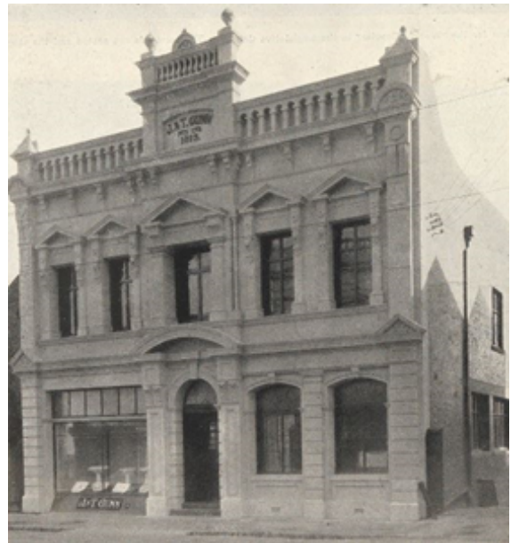
J & T Gunn building as rebuilt following fire - May 1931 Weekly Courier 15 July 1931
