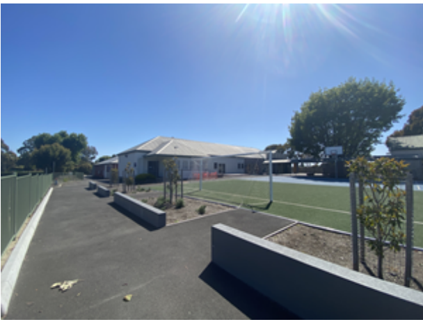
Rear elevation of main 'C' shape building Heritage Tasmania
