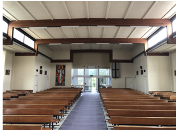
Within the nave, looking westwards towards the narthex and its three floor-to-ceiling windows. © DPIPWE 2019
