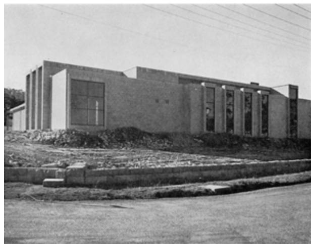
c.1967: from the south-west, at the corner of Bay Road and the Esplanade. R Farrington
