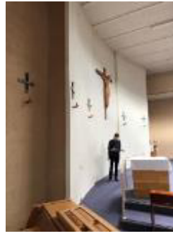
The reredos' concave surfaces viewed from the nave's north-east corner. © DPIPWE 2019
