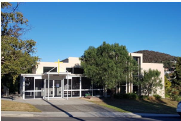
Church of the Incarnation from the west. Monsignor Rogers' grave is to the right of the doors. © DNRET April 2022
