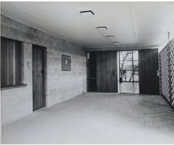
c.1967: Pre-Narthex, looking south. Bookstall servery hatch and access door are at left. R Farrington, courtesy of Paul Johnston
