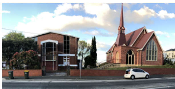
St Stephen's Hall and Church DPIPWE, 2020
